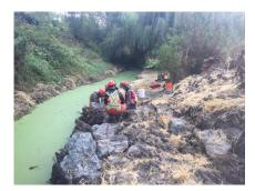
Working with the Public Works Creeks & Waterways crew, a large section of Swan Creek (off Columbine) has had significant work done to increase flow and improve the habitat for fish spawning. Several yards of spawning gravel was placed in the creek bed plus a small section of large boulders and stumps were added
